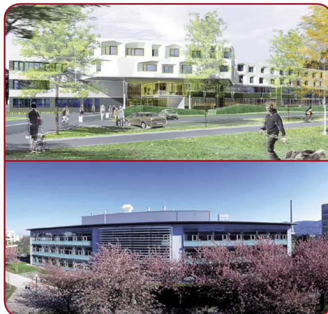
Current (bottom) and future (top) National Center for Tumor Diseases (NCT) building in Heidelberg.
